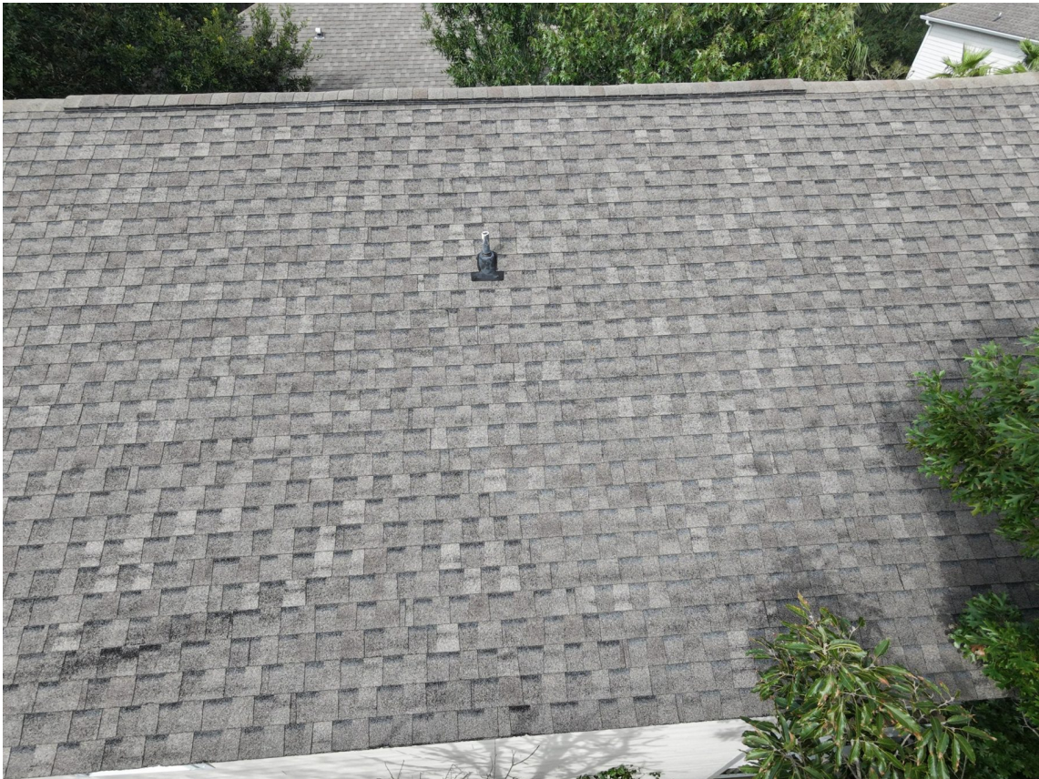
Figure A: Main roof slope overview — representative of overall condition
